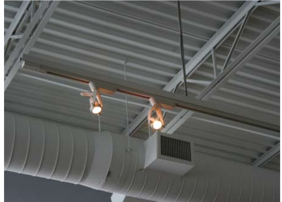
Track lights with open-web joists.
