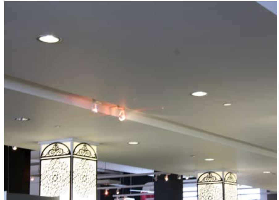
Down lighting in bulkhead.
