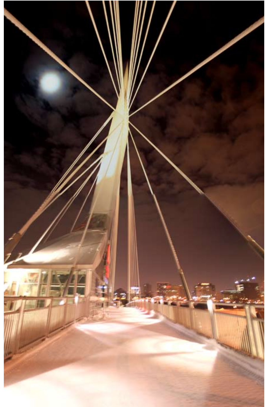
Cable stays and mast lighting.
