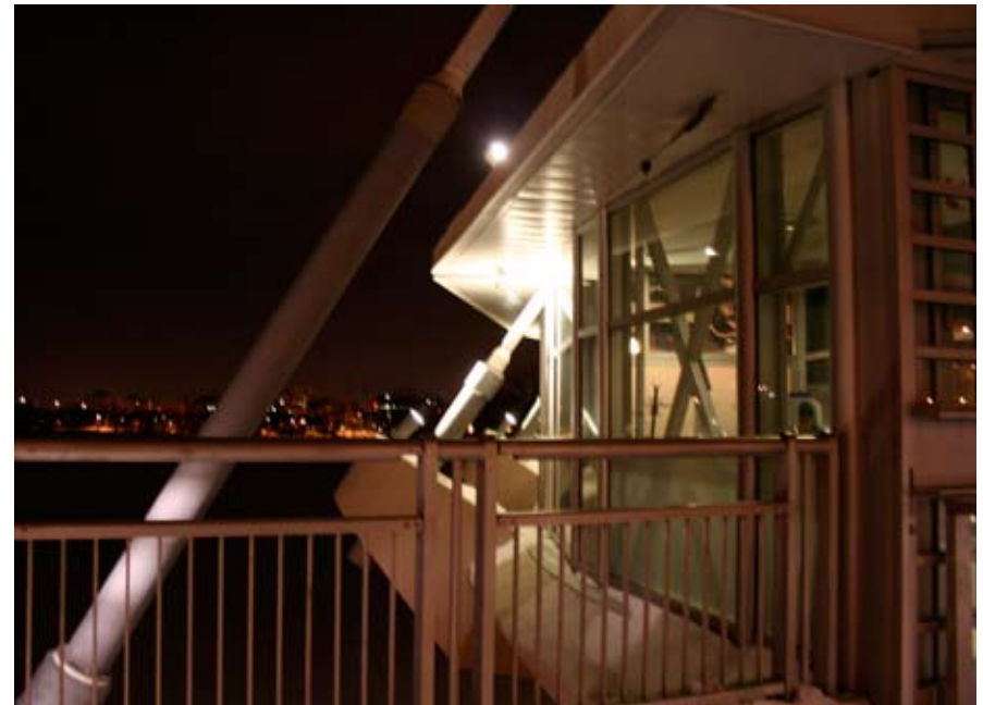
Yard lights for bottom third of mast.
