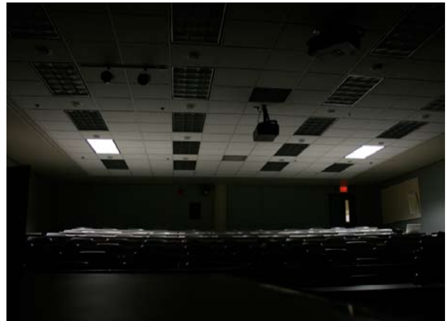
Controllable banks of fluorescent fixtures.
