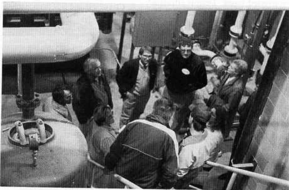
Touring the Pound-Maker Ethanol facility
