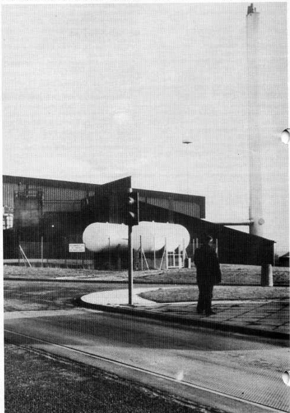
The Byker mechanical separation plant in northeast England, which now has six years operating experience.
