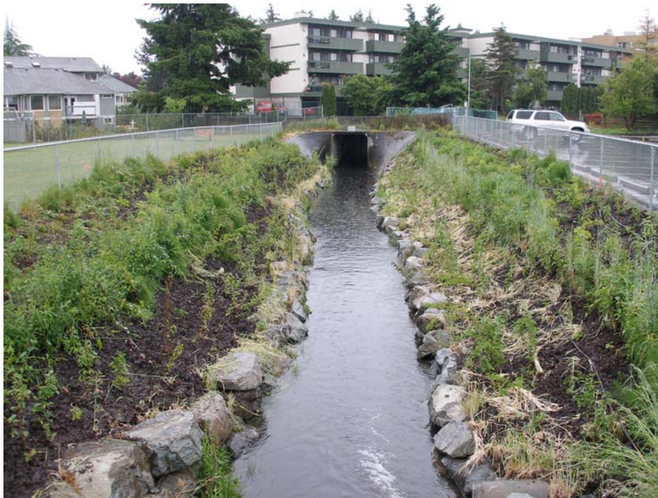
Looking east from middle of bridge
