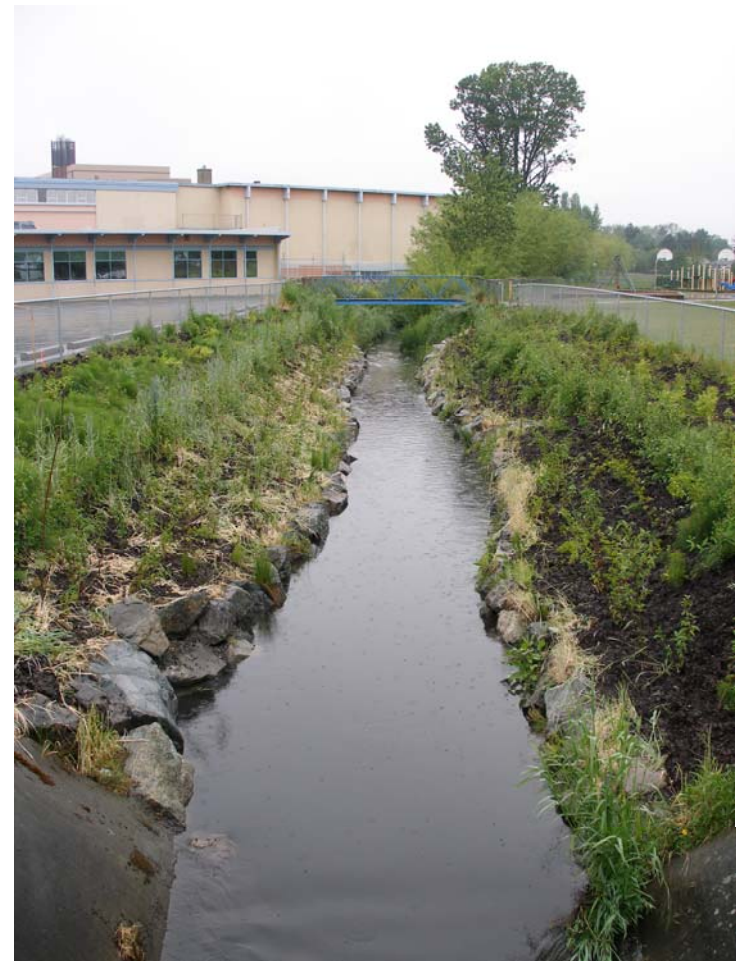
Looking west from top of culvert
