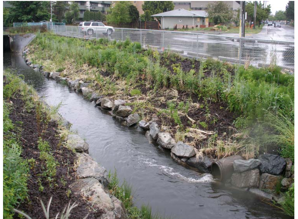
Looking east along south side
