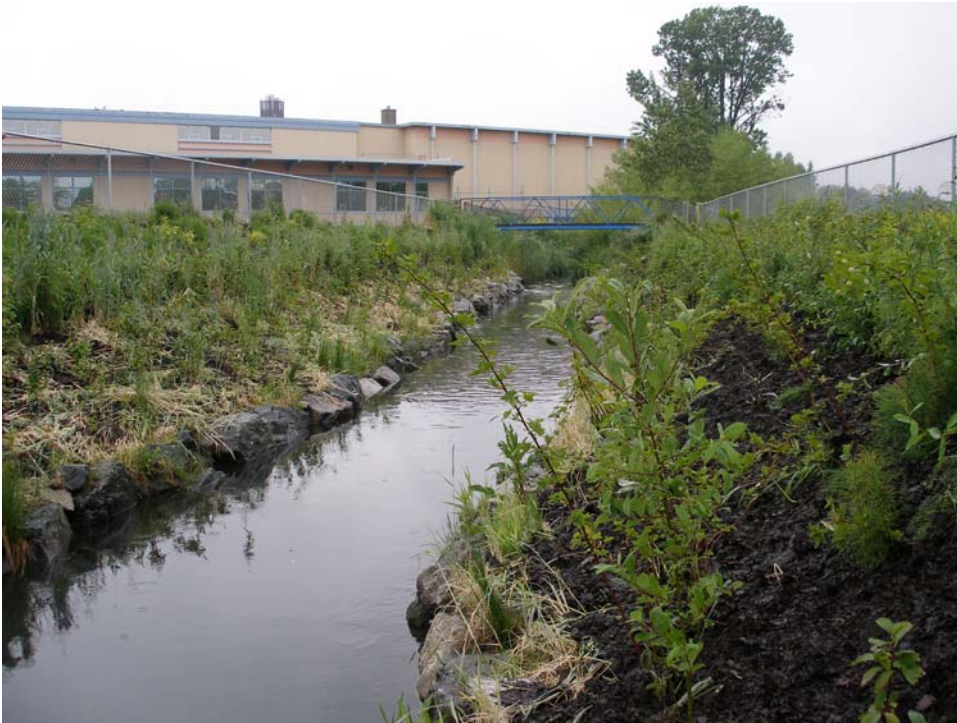
Looking west along lower slope, north side
